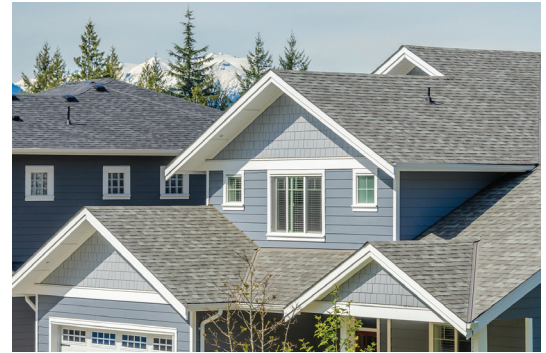
Asphalt Shingles
