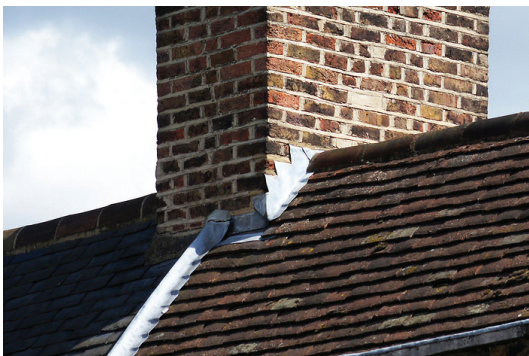
Roof Flashing
